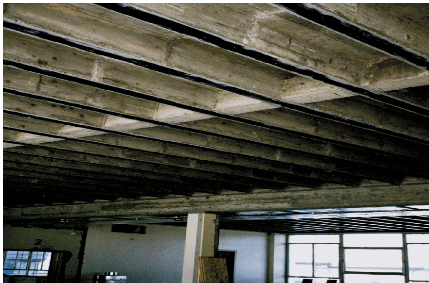
"Build Strip HS" Installed at Reinforced Beam
